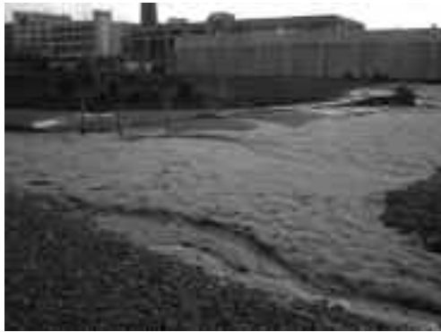
Before – Surface runoff picks up speed over non-vegetated areas and carves out channels.
