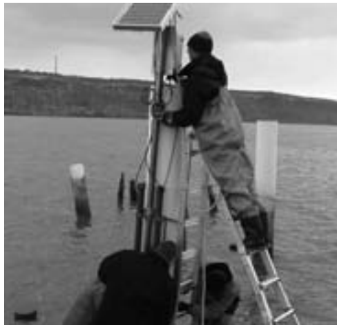
Positioning the equipment
